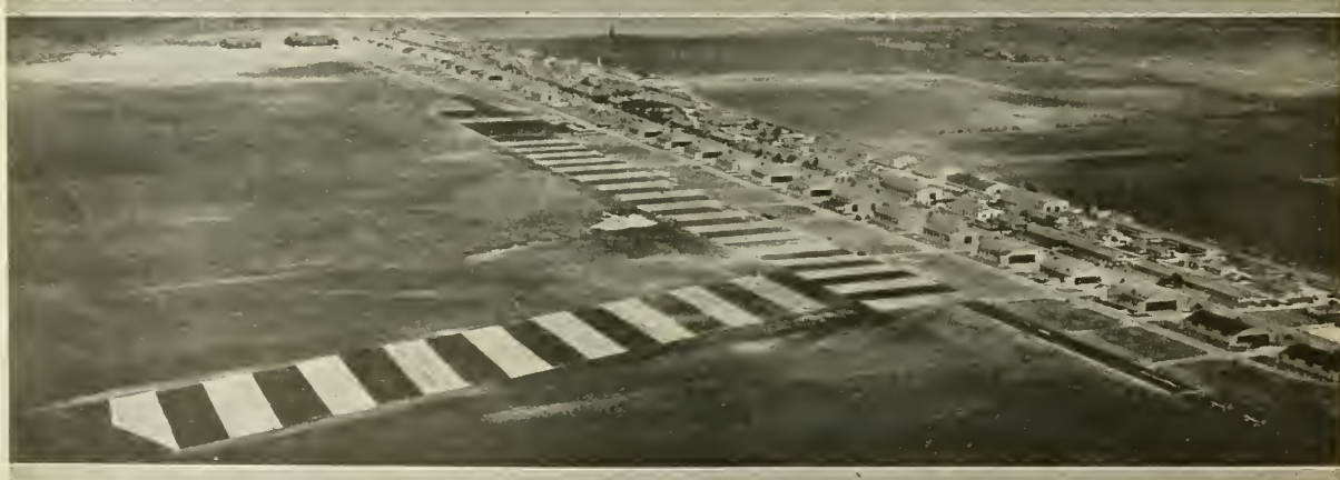
New striped runway system at the Army training base, Kelly Field, San Antonio, Texas
